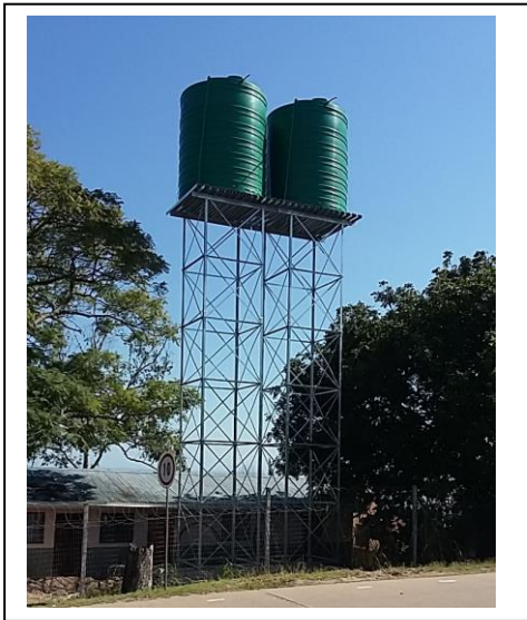
Water tanks giving back up supply of water, & Care Workers' Office
